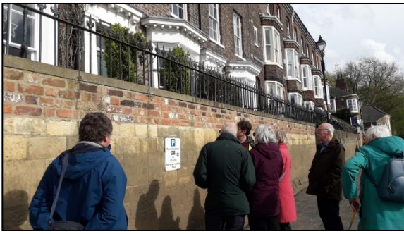
Raised flood wall in front of houses near King's Staithe
