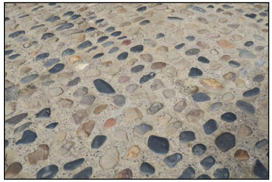
Variety of cobbles at Queen's Staithe [Simon Green]
