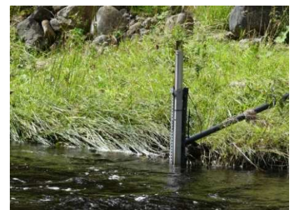
One of Zora's river level measures, which can store two months' data
