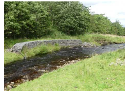
A section of bank reinforced with gabions to prevent erosion
