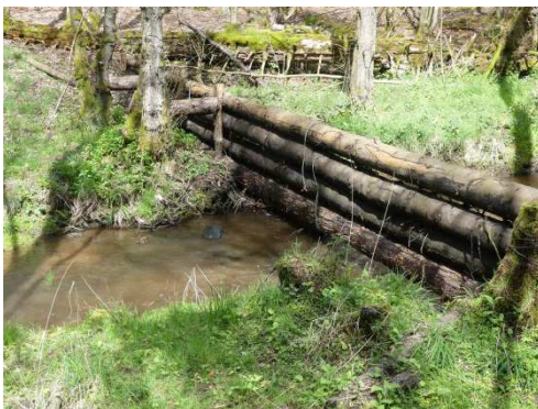
One of the woody dams. Note the gap between the level of water at the time of our visit and the bottom of the dam. In flood events, the dam will encourage water to spread out over the adjacent floodplain, thus slowing its flow downstream
